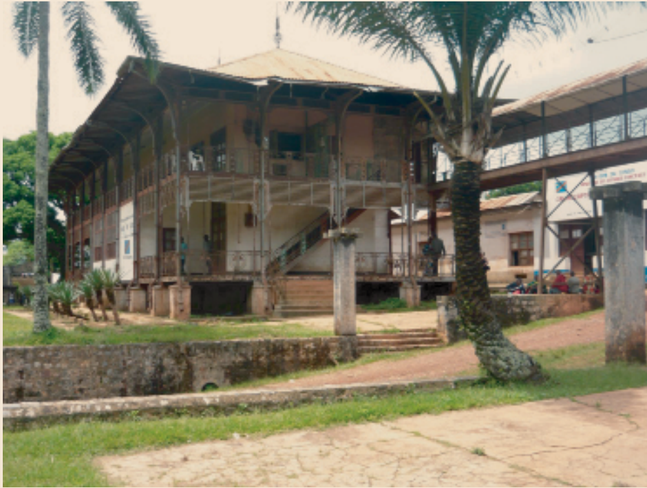
Fig. 6. Hôtel ABC in Mbanza Ngungu, built between 1904 and 1908 out of prefabricated metal components imported from Belgium. Source: photograph Johan Lagae, 2009.
