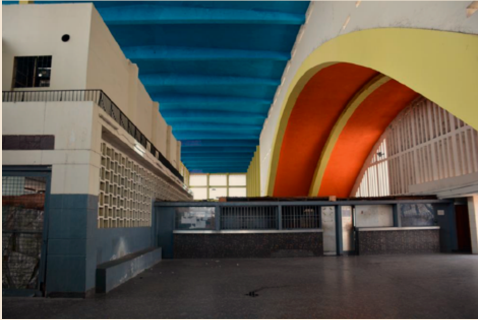
Fig. 8. Interior of the Gare Fluviale in Kinshasa, designed by architect Jacques Delire, 1956-1959. Source: photograph Johan Lagae, 2017.
