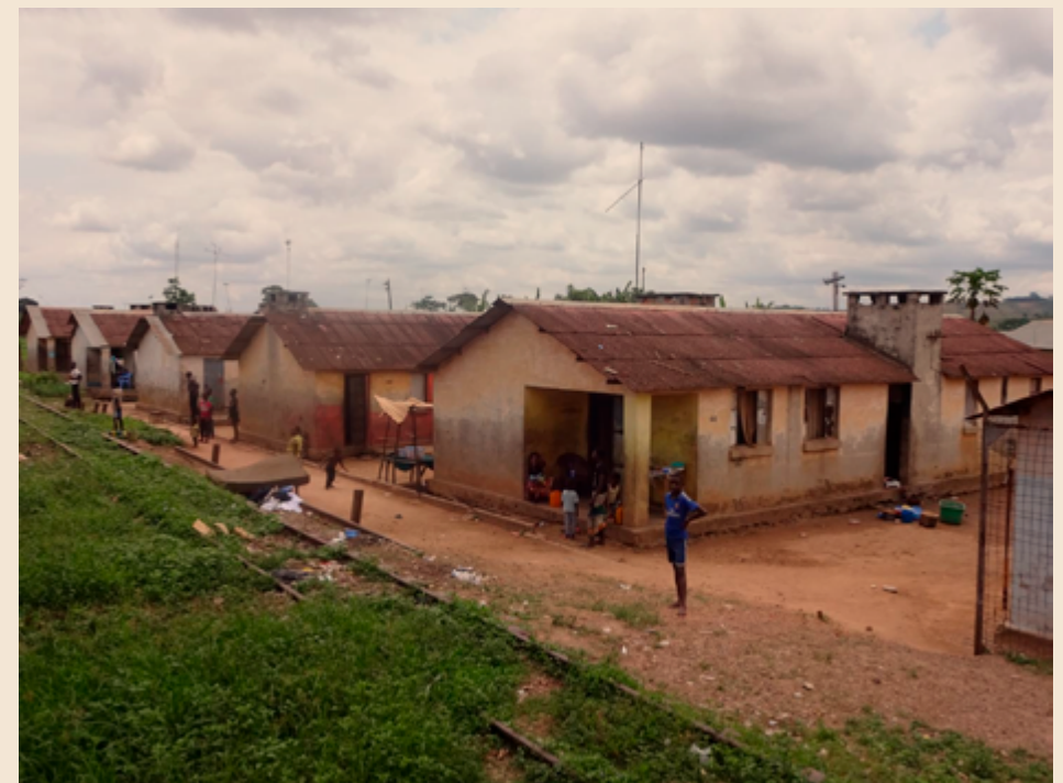
Fig. 11. The OTRACO workers’ camp in Kisantu. Source: photograph Johan Lagae, 2015.
