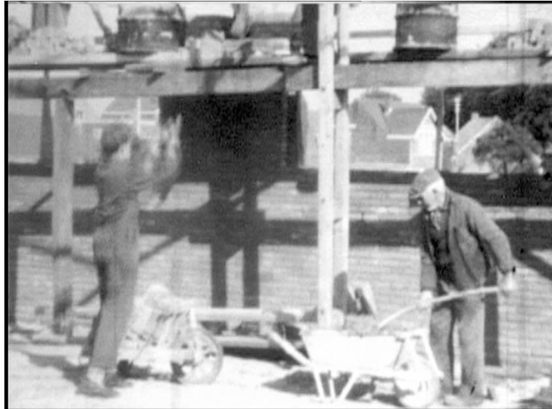
Figure 4. A man tosses bricks to a worker on scaffolding, while another throws mortar into a bucket. Photo: Ginderbuiten 1955: bouw en inwijding van de Noodkerk.
