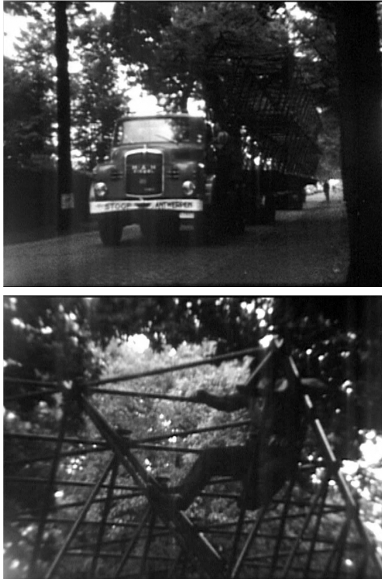
Figure 6-7. The steel space frame was delivered by truck, with its workers sitting on top.
