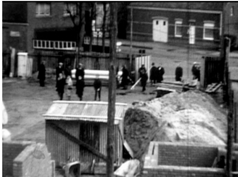
Figure 10. As the gates opened for the church's inauguration, the construction site briefly became a place of public gathering. Photo: Ginderbuiten 1965: Bouw en inwijding van de Nieuwe Kerk .
