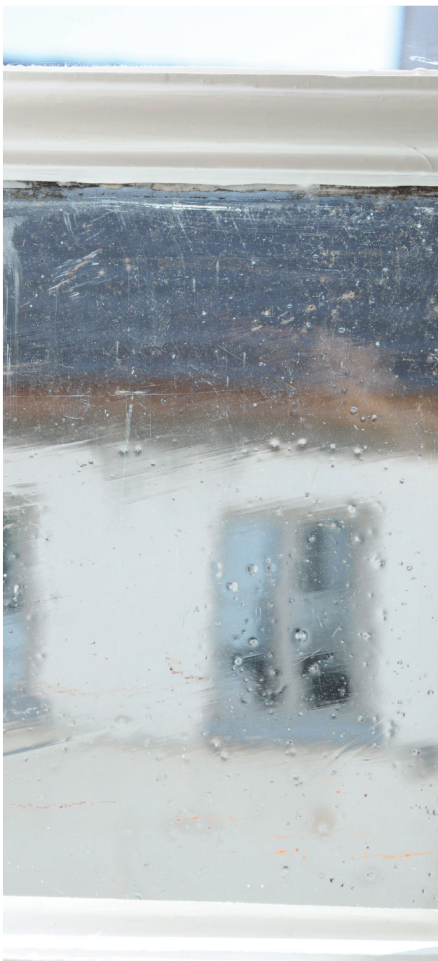
A pane of cylinder glass, in one of the rooms of the first floor of De Neve-d'Hanins House. © Liesbeth Langouche.
