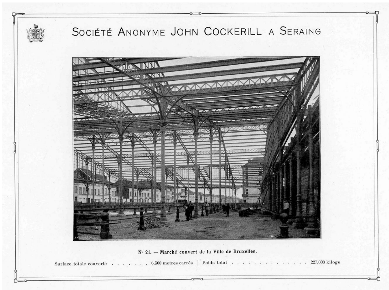
Figure 3: The relocation of the metal hall in front of the Brussels slaughterhouse complex was documented in S.A. John Cockerill's company catalogue. (Société Cockerill ca 1910, MMIL)
